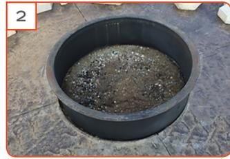
**STEP 2** - Place and center steel ring on prepared base.
