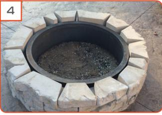
**STEP 4** - after placing blocks around the ring, adjust the blocks in or out to make circle fit tight.
