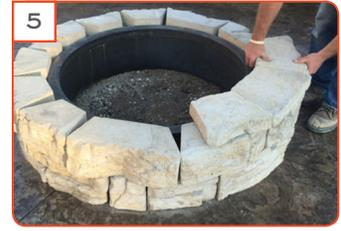
**STEP 5** - place caps in circle around fire pit. Adjust the caps in or out to make them fit tightly together.
